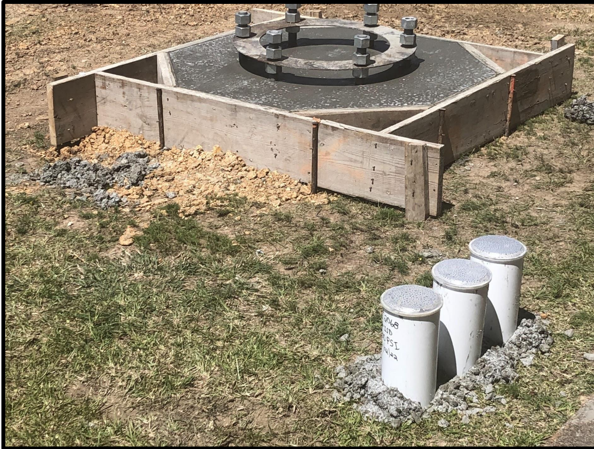
Radio Tower Foundation
